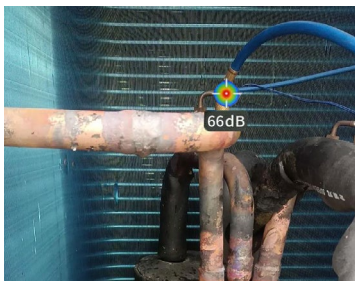
Compressed Air System Leaks
