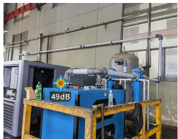
Compressed Air System Leaks
